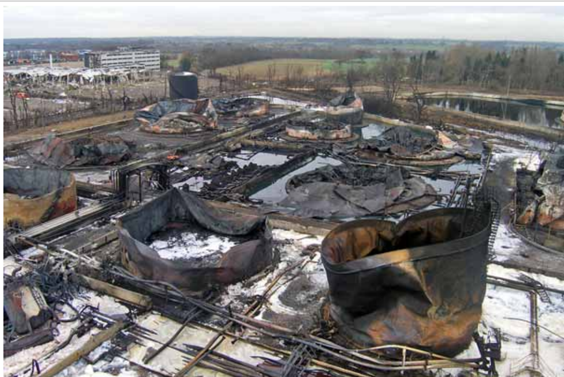
Figure 19 Devastated tanks after the fires © Hertfordshire Constabulary
